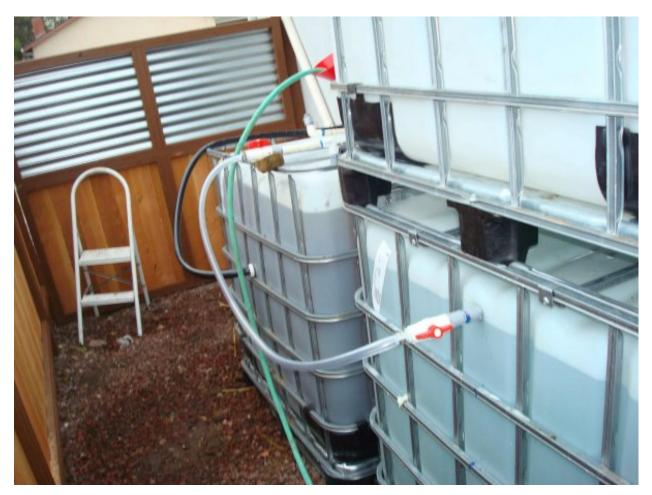
Figure 29. Figure showing how gas is piped from digestor to collector
