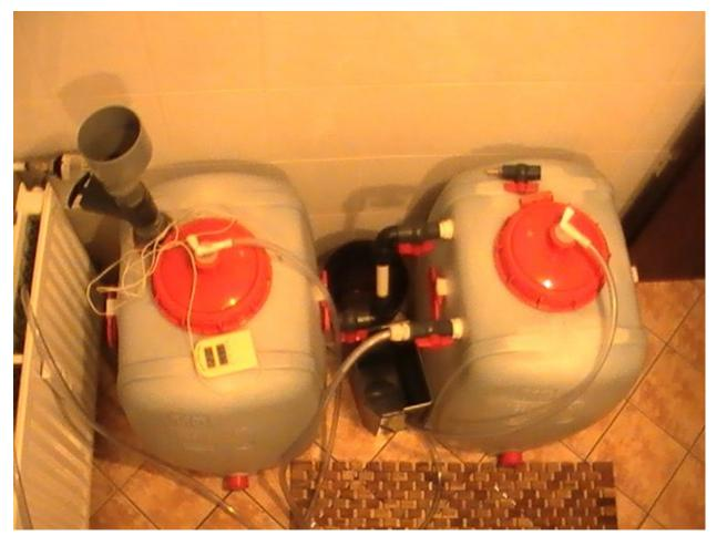
Figure 26. In the Culhane's upstairs bathroom in Germany a two chamber biodigestor made from 110 liter beer fermentation tanks takes their baby's diaper wastes and turns it into cooking gas and fertlizer. The system was started with baby fecal material only and once it started producing flammable gas left over baby food was used to dramatically increase production. This experiment proved that biogas could be done without odor or problems indoors using only wastes found in the average home.
