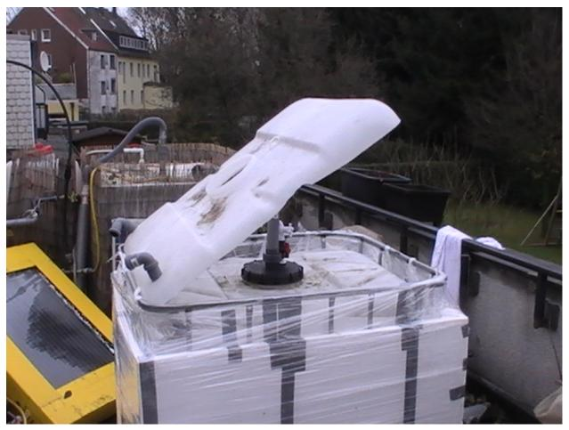
Figure 24. The Culhane's second family size biodigestor is made from a 700 liter IBC tank nested inside a 1000 liter IBC that is insulated with styrofoam. Hot water discharged from baths and showers surrounds the internal tank and keeps the bacteria at their desired temperature.
