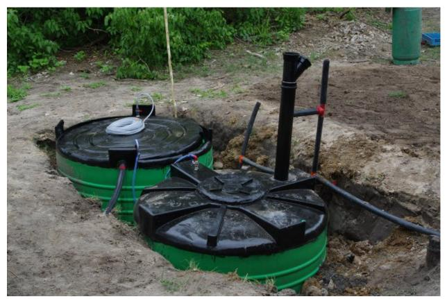
Figure 45. Where the Selinda system called for a 5000 liter primary tank because of the volume of kitchen waste, we only needed a 2500 liter tank for the Zarafa lodge. The difficulty in both cases is sealing the lid so that it doesn't crack and leak. Heat welding seems to work with some tanks; in Kenya the lid is made of a different plastic and won't weld properly.
