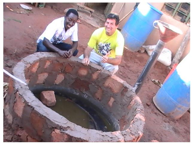
Figure 37. An ARTI style digestor with the primary tank made of cement and brick sunken into the ground and a 1000 liter inverted water tank as the gas holder; this solution is advisable when tanks are more expensive or difficult to obtain than cement and brick. The digestor need not be submerged – this only adds to the difficulty of making it because of the labor required to dig, but it does allow for eventual connection to an Insinkerator for gravity feeding.
