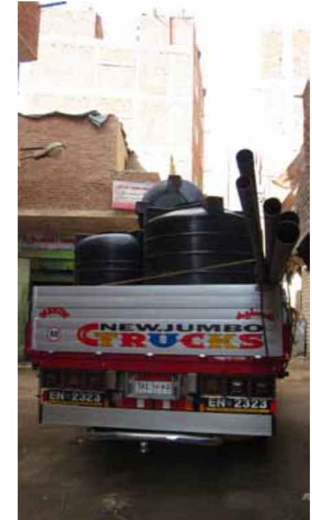
Fig.5_03: Transferring the equipments to the site in Ezbet Al-Nasr
