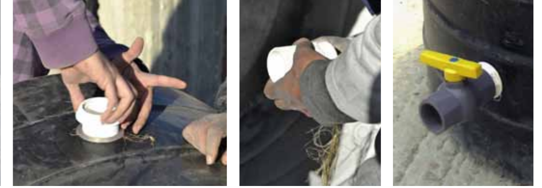
Fig.I_11: Then install the PVC valve
