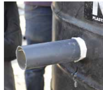
Fig.I_13: Then fix the 2"-2.5" pipe
