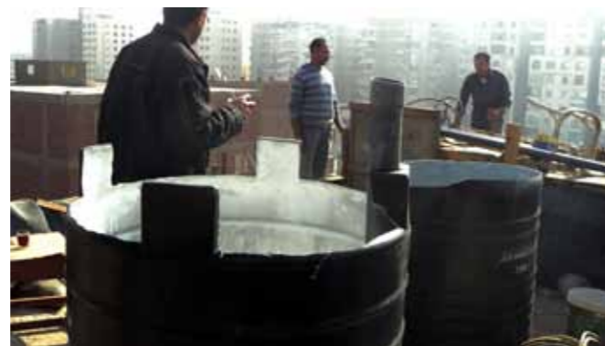
Fig.5_17: STEP 06 _Cutting the top of both tanks (taken by: Heidi Fink)
