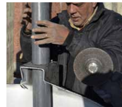
Fig.I_08: Insert the pipe to make sure of the hole width, then fix the L-shape fitting and then re-install it again
