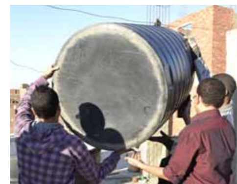
Fig.I_16: Turn the smaller tank upside down
