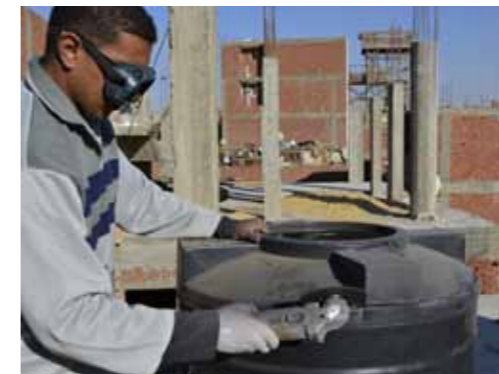
Fig.I_04: Use the automatic saw for cutting the top of both tanks
