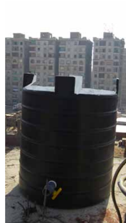
Fig.5_21: STEP 07 _Installing the emergency (to empty) out-let pipe
