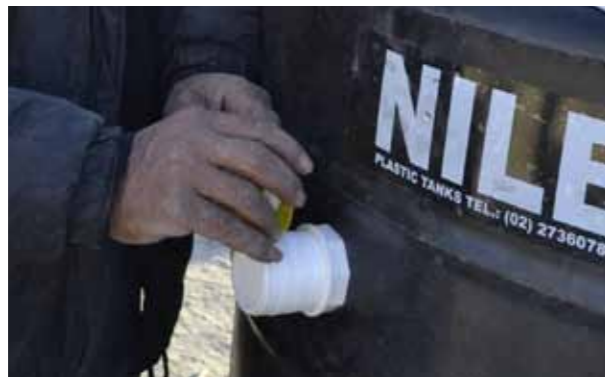
Fig.I_12: Cut another upper hole from another side of the same tank (the bigger one), then install the fittings, do not forget to use the suitable needed PVC cement and adhesive tapes
