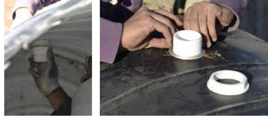
Fig.I_10: Fix the 2" fitting using the needed fibers
