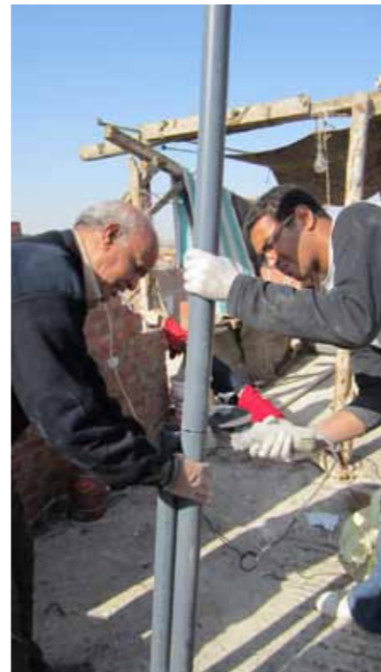
Fig.5_20: STEP 06 _Preparing pipes for the installation of the in-let and out-let holes
