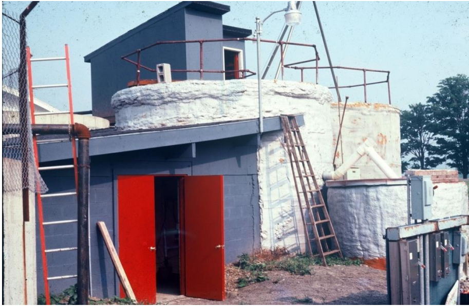
Research digesters, Cornell, ~1977
