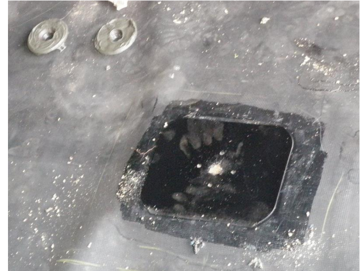
Flanges for Dickinson EPDM digesters
