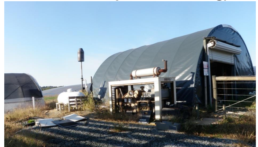
Engine-generator (inoperative due to inadequate scrubbing)
