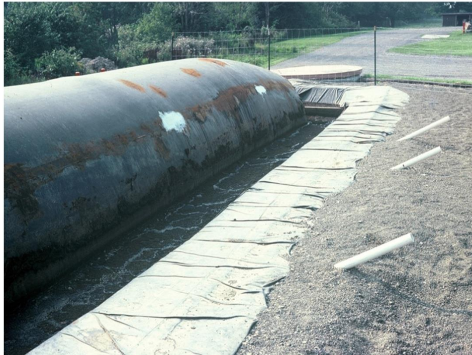
Figure 4. Plug flow digester
