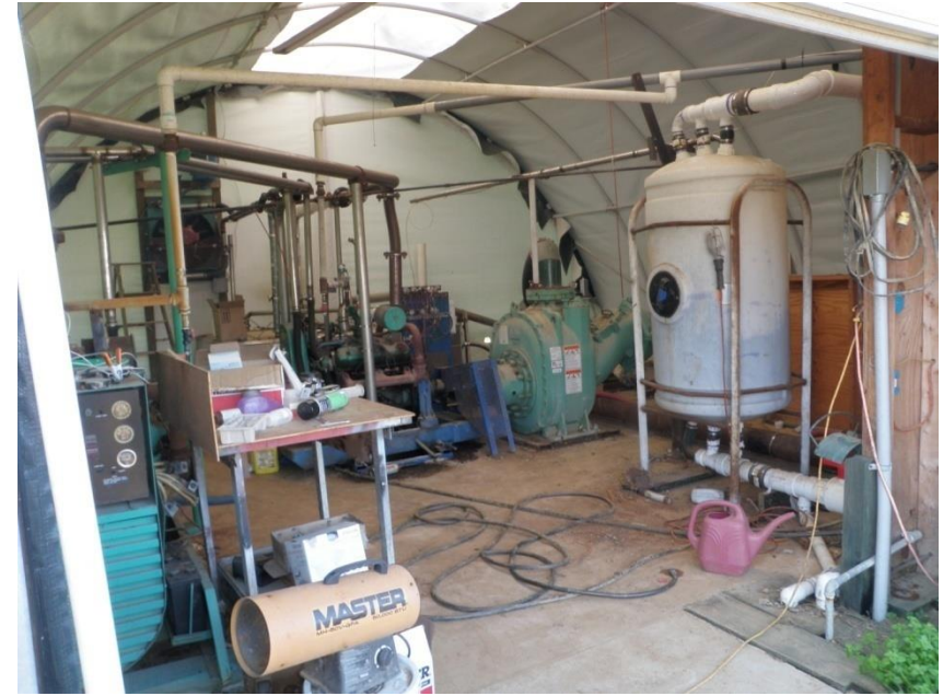
Engine-generator (inoperative due to inadequate scrubbing)
