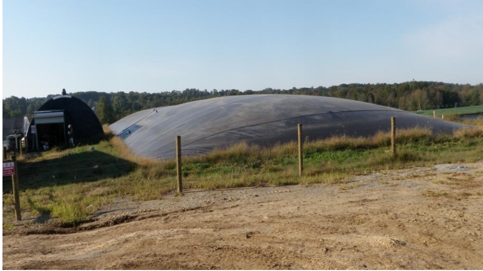
Covered lagoon and operations shed
