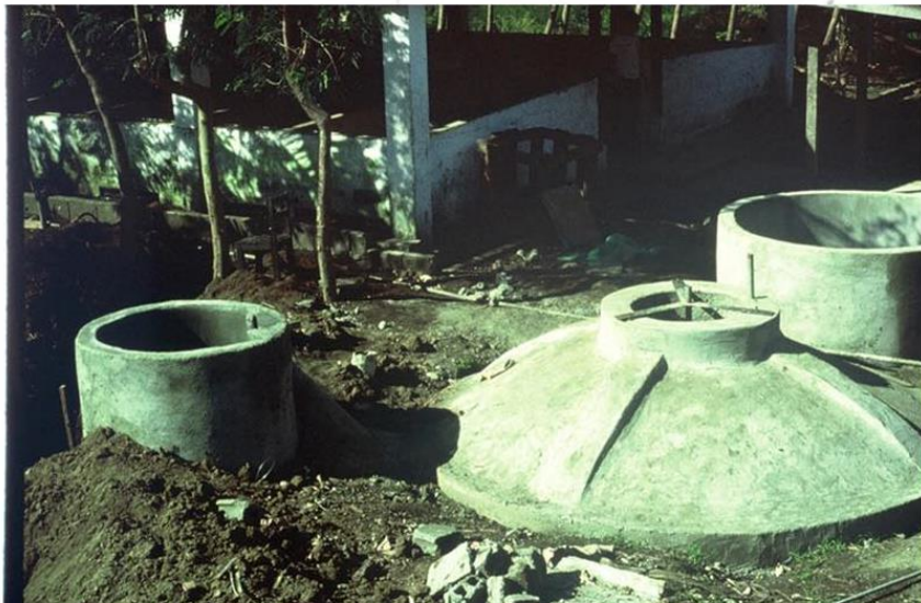
Concrete construction in the Philippines, 1985
