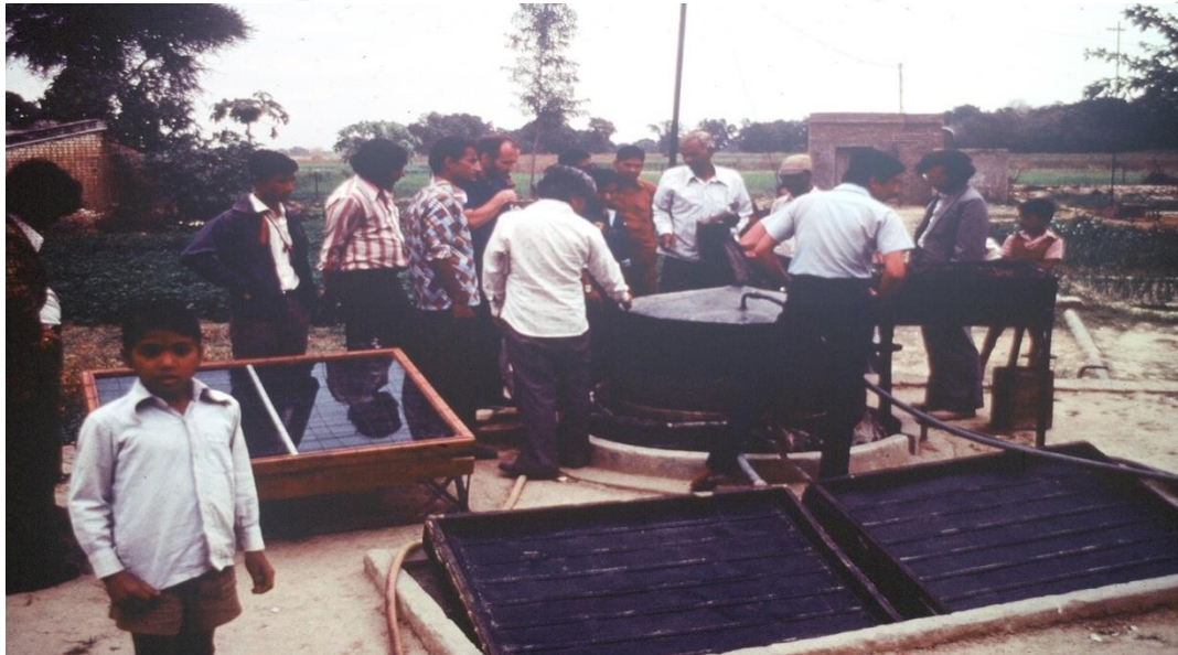
Figure 2 Floating cover (Indian) digester
