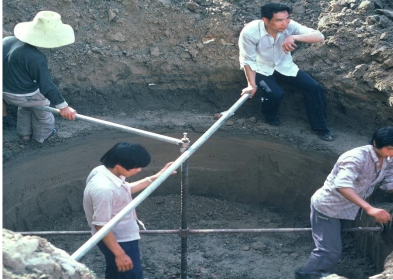
Steel frame set for pouring dome
