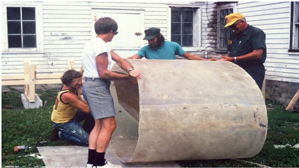
Fiberglass digester construction at Rutan Biogas Workshop, ~1978
