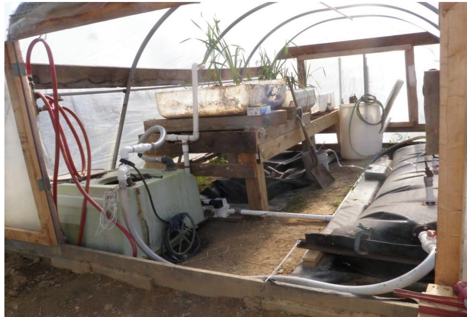
Pieces In place
