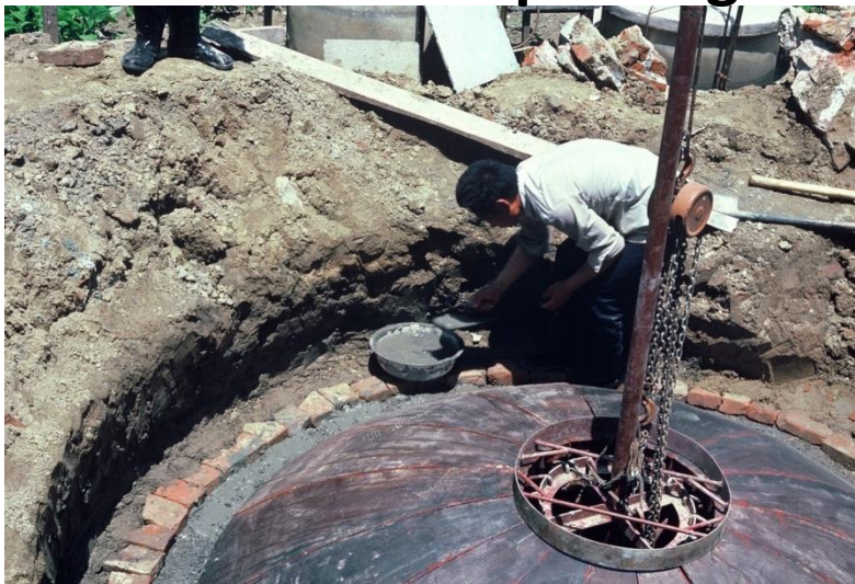
Steel frame set for pouring dome
