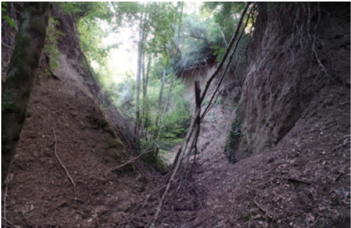
erosion caused by rainwater runoff
