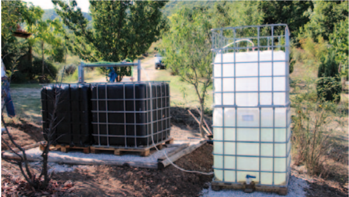
New built Biogas Digester and Gas Storage at Skala
