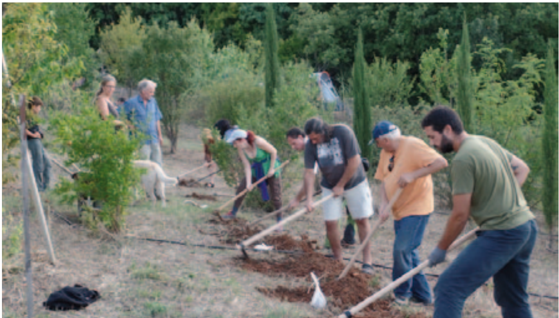
Building a swale in the orchard
