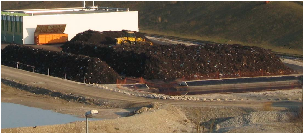
Figure 8.1-27: Post-composting of the digested sludge, in open windrows
