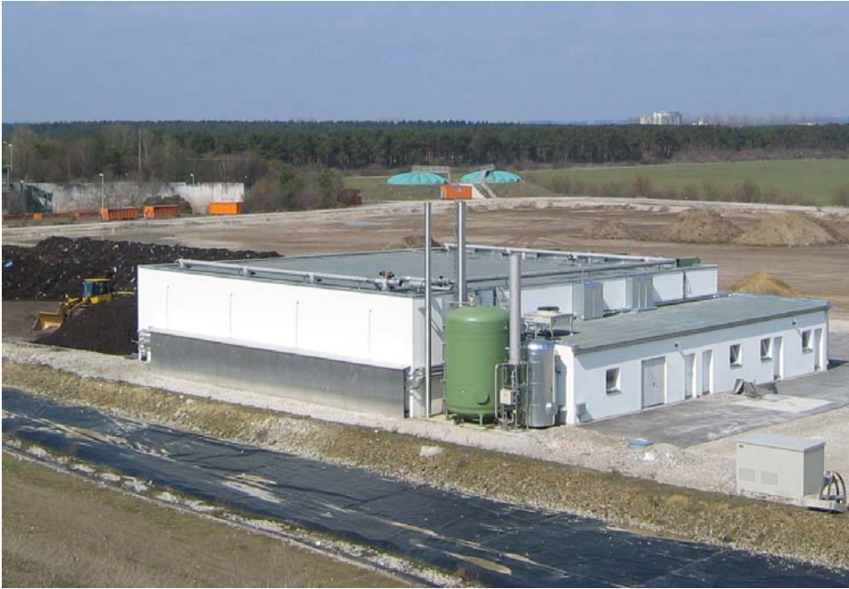
Figure 8.1-24: Biogas plant from BEKON, Munich
