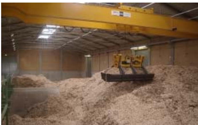
Figure 3.2-2: Crane system in operation 9
