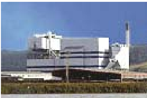
Figure 8.2-8: Biomass combustion plant Glanford
