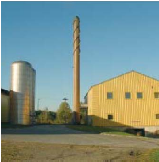
Figure 8.2-2: Straw combustion plant Schkoelen
