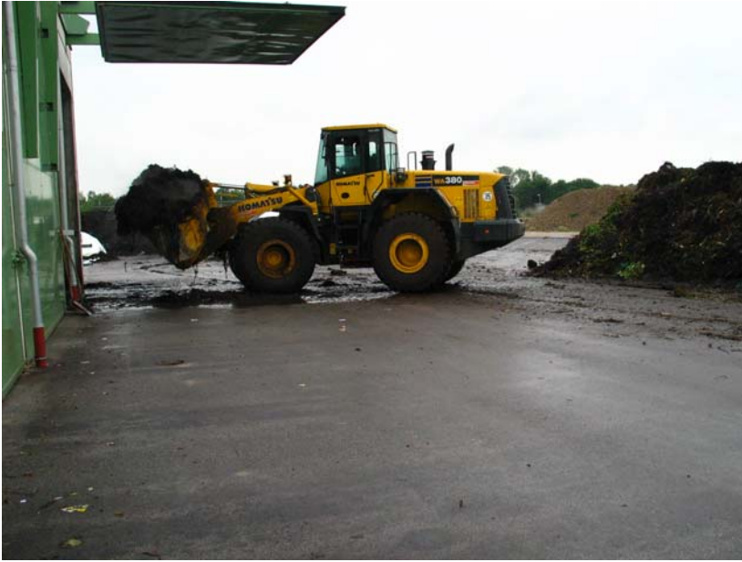
Figure 8.1-26: Wheel loader in the process of loading the digester/ reactors
