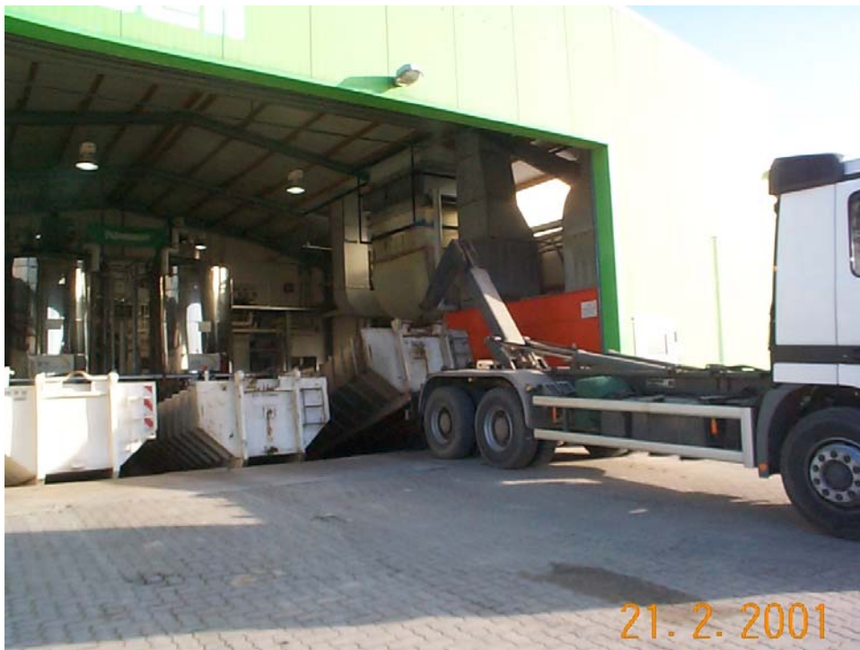
Figure 8.1-19: Substrate reception area, with sanitation units (behind)
