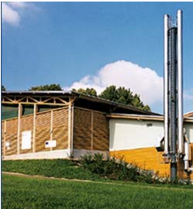
Figure 8.2-1: Biomass combustion plant in Dresden
