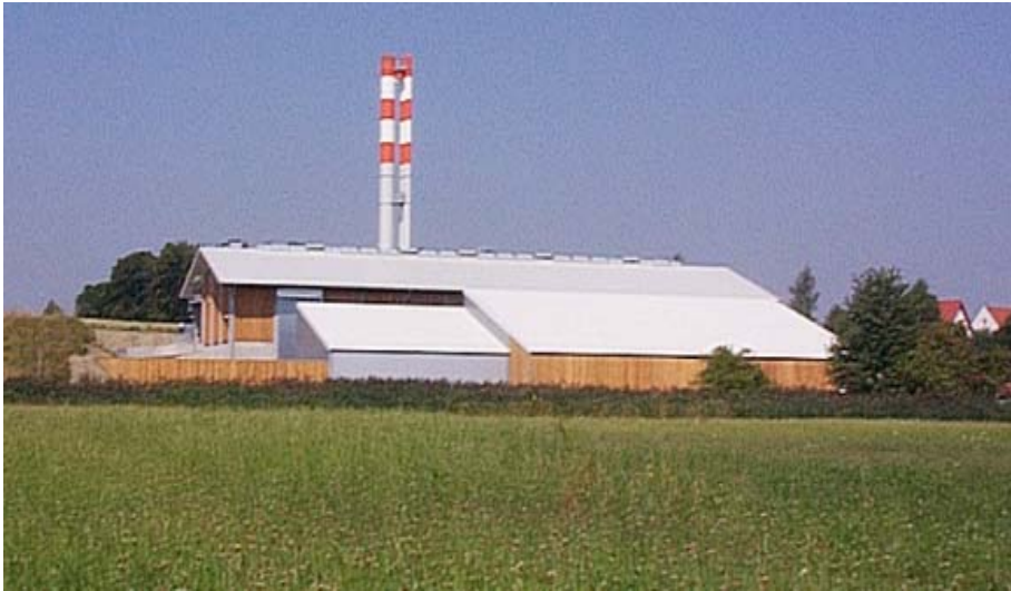
Figure 8.2-5: Biomass combustion plant Pfaffenhofen
