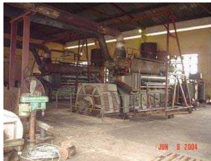
Figure 7.1-1: Power generation on Phu Quoc island: New power plant near the capital Duong Dong a-Diesel generators at the old generation site
