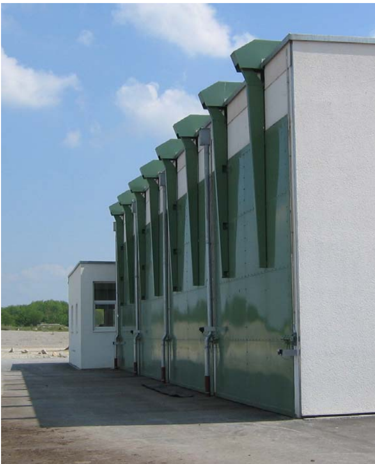
Figure 8.1-25: Closed tunner reactors for dry fermentation
