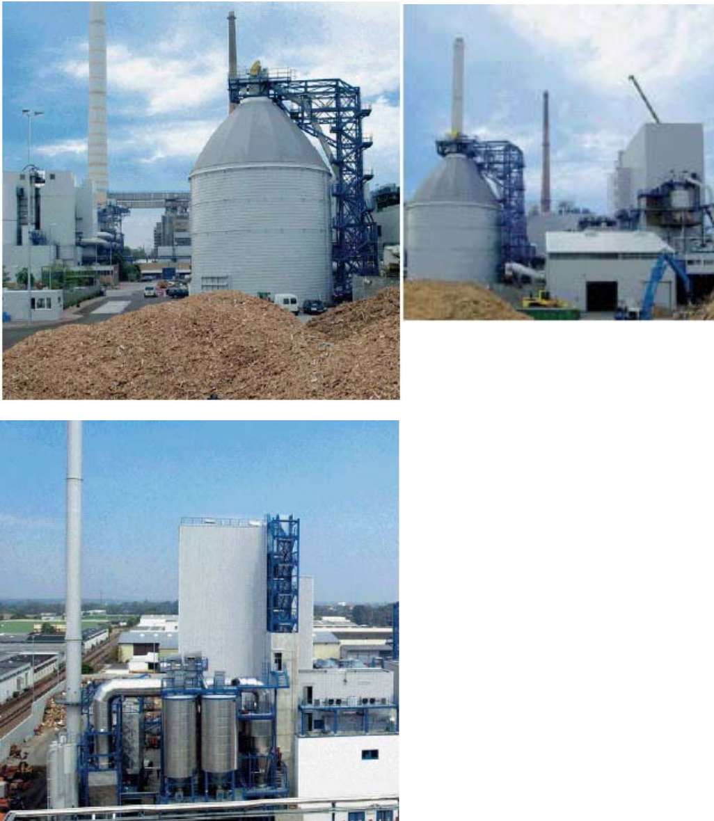
Figure 8.2-6: Biomass combustion plant Mannheim
