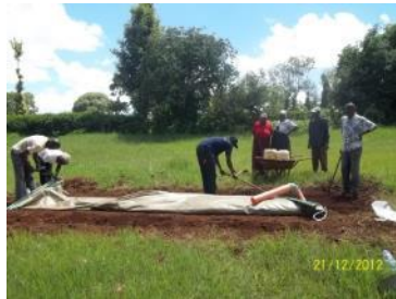
Laying the envelope
