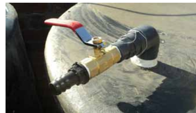
Fig.5_24: Installing the valve after the filling (taken by: Heidi Fink)
