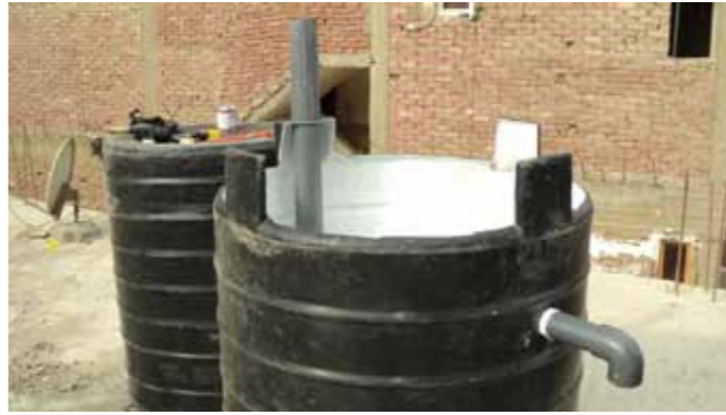
Fig.5_17: STEP 07 _Preparing for installing the in-let and the out-let pipes in the bigger tank (taken by: Heidi Fink)
