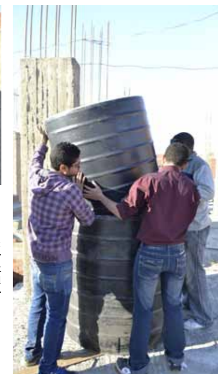
Fig.I_17 (to the left): Put it inside the bigger tank, after filling the tank with dissolved dung and water
