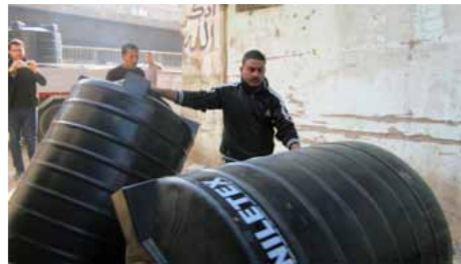
Fig.5_07: Tanks are moved to the first house to start the installation
