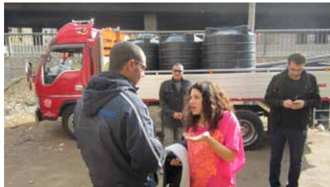
Fig.5_06: Tanks, equipments and all materials arrived to the site
