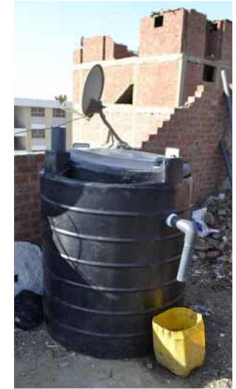
Fig.5_31: The Biogas unit is ready, should be left for four weeks in winter times until it produces the biogas (the upper smaller tank should rise up as an indicator that the unit started to produce the gas)
