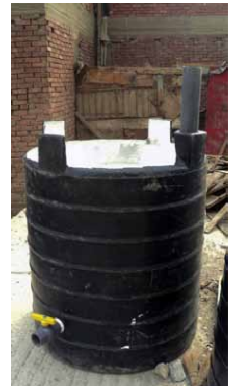
Fig.5_21: The bigger tank after installing the in-let and the emergency out-let pipes (taken by: Heidi Fink)
