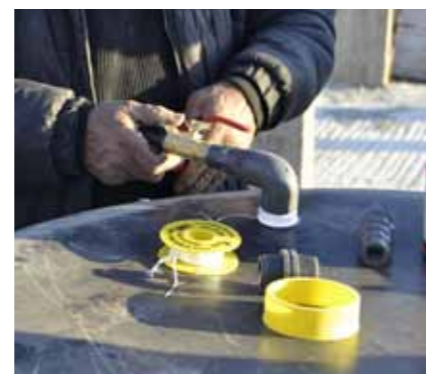
Fig.I_15: Cut a third hole, this time, at the bottom of the smaller tank (for the gas exit), use the same materials as before
