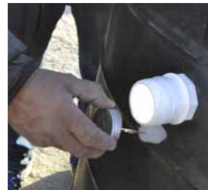
Fig.I_12: Cut another upper hole from another side of the same tank (the bigger one), then install the fittings, do not forget to use the suitable needed PVC cement and adhesive tapes
