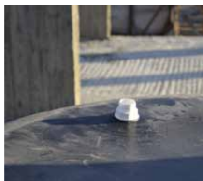
Fig.I_15: Cut a third hole, this time, at the bottom of the smaller tank (for the gas exit), use the same materials as before
