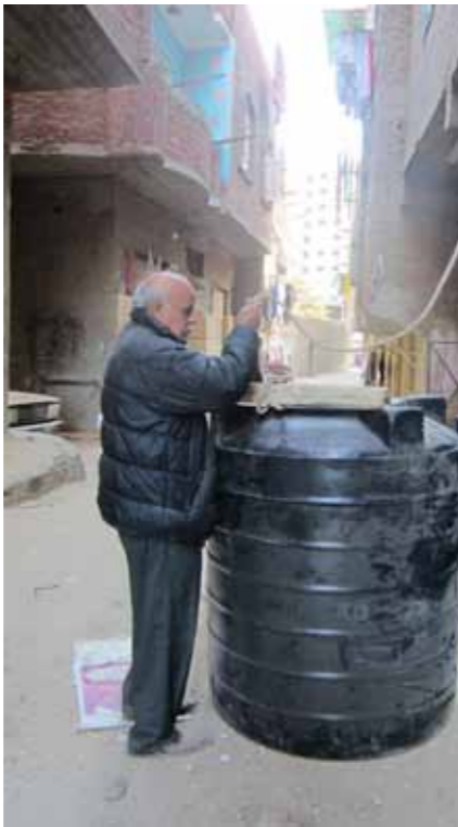
Fig.5_15: STEP 05 _The start, lifting the tanks to the rooftop using a wooden rod and a long rope
