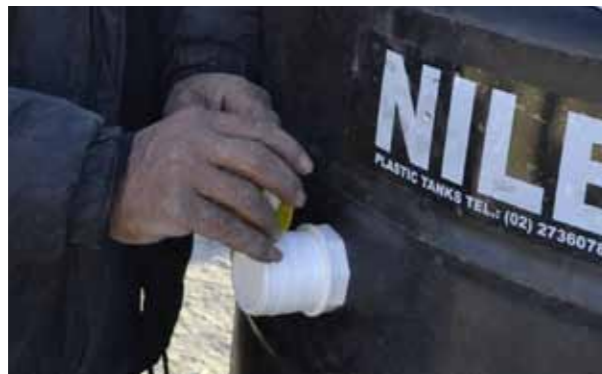
Fig.I_12: Cut another upper hole from another side of the same tank (the bigger one), then install the fittings, do not forget to use the suitable needed PVC cement and adhesive tapes
