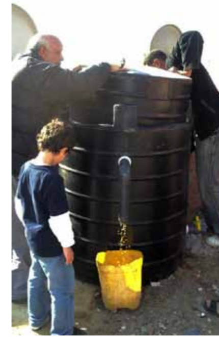
Fig.5_30: STEP 12 _Puttin the smaller tank above the bigger one (upside down) (taken by: Heidi Fink)
