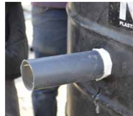
Fig.I_13: Then fix the 2"-2.5" pipe
