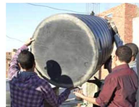
Fig.I_16: Turn the smaller tank upside down
