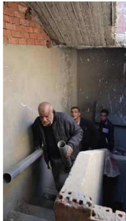
Fig.5_19: Moving the pipes and other small equipments through the staircase
