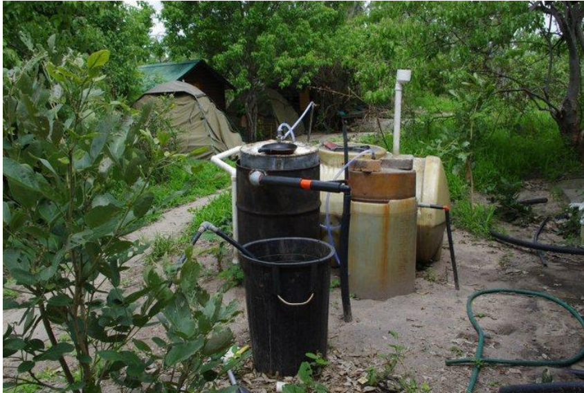
Figure 18. Photograph of small-scale digester built at Selinda Camp.
